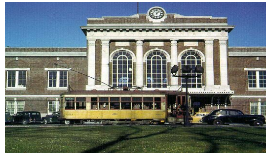
Figure 8 - A good connection to rail service is essential.
