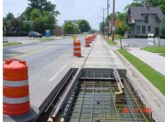
Figure 15 - Completed section of track.
