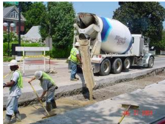
Figure 13 - Base concrete pour from adjacent lane.
