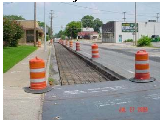
Figure 14 - rebar grid installed ready for track.
