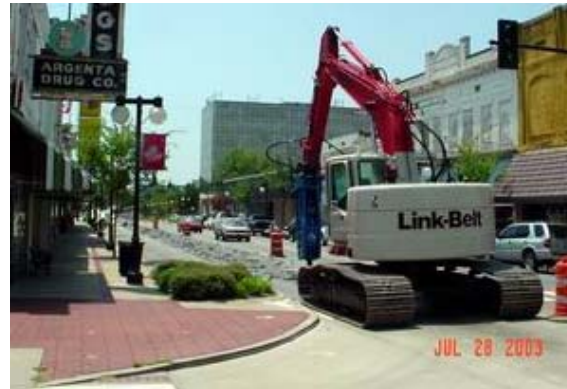
Figure 12 - Work zone set up and street excavation in Little Rock.
